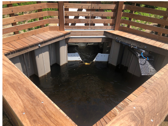
Resting pool at the top of Woodhull Dam fish passage. Photo credit: Valerie Virgona, Peconic Estuary Partnership
