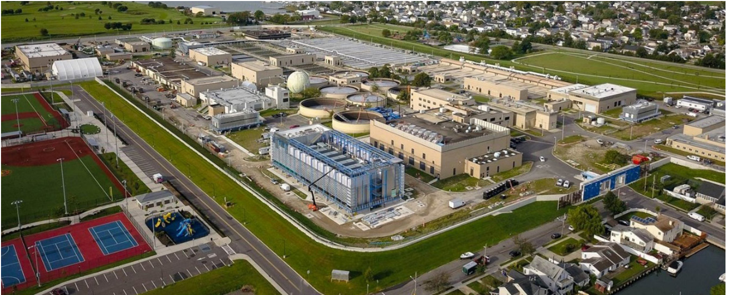
Aerial view of the South Shore Water Reclamation Facility, Nassau County, NY. Photo credit: Veolia North America
