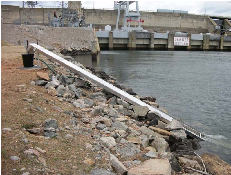
South Eel Trap 12.8M long and sits at a 38 degree angle 151L holding tank with flow through
