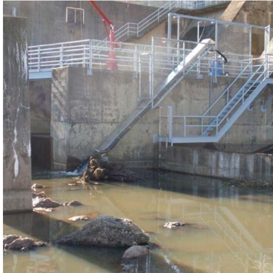
South Eelway 8M long, 41 degree ramp angle 265 L holding tank with flow through
