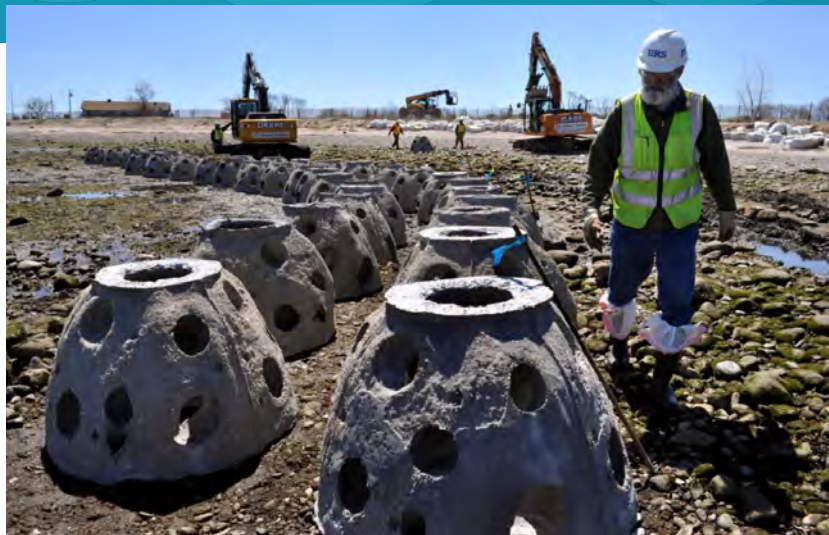
Figure 15. Precast concrete reef balls called Pallet Balls being deployed at the Stratford Point Living Shoreline in 2014. Photo credit: CT DEEP.
