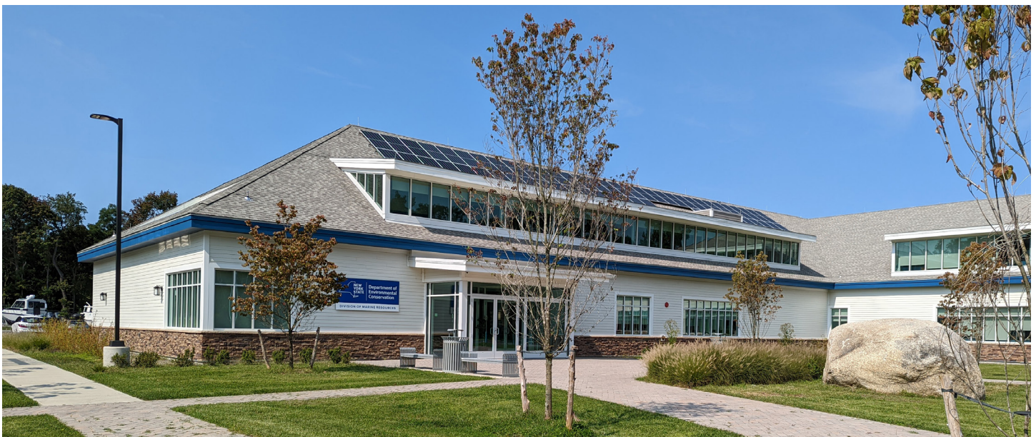
The new headquarters of NYSDEC's Division of Marine Resources located within Nissequogue River State Park, Kings Park, NY. Photo credit: Alexa Fournier, NYSDEC
