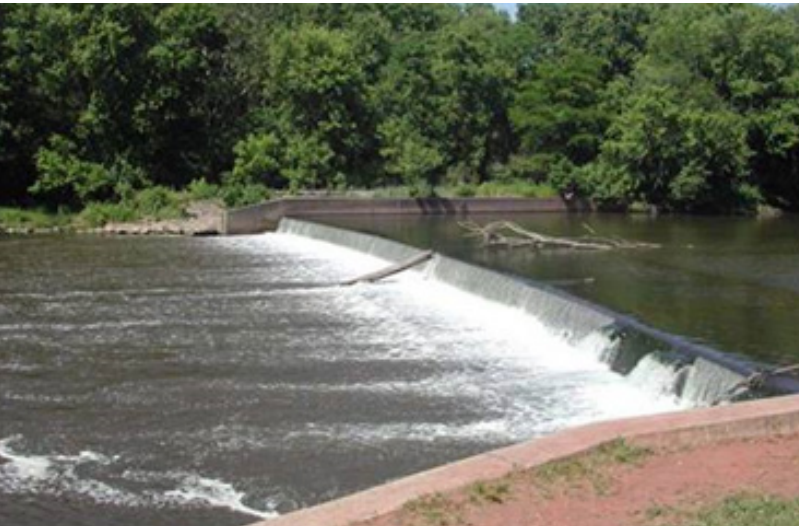
Headgates Dam. Photo credit: NOAA
