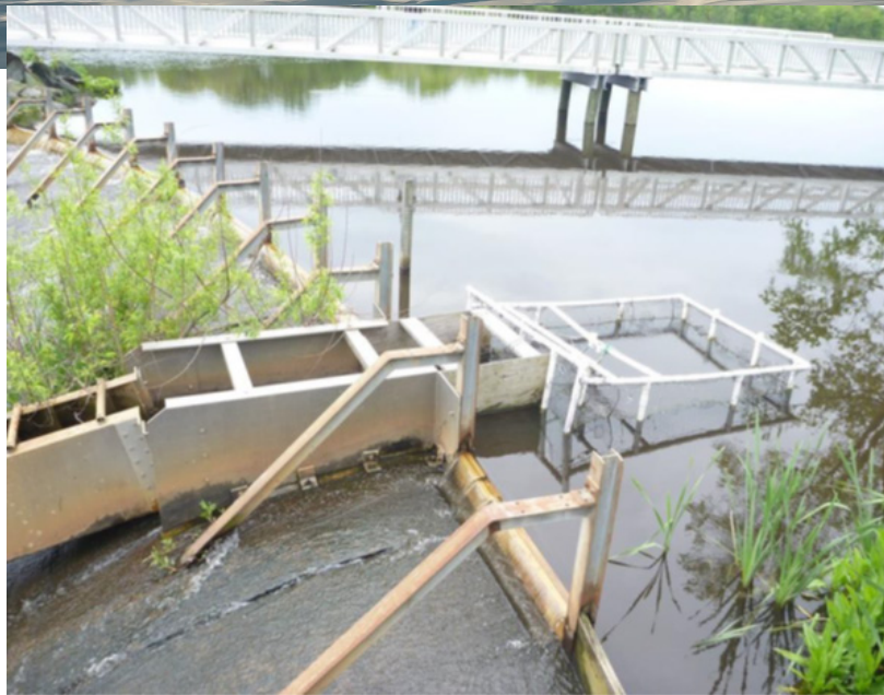
A fish ladder and exit trap at Garrison's Lake, north of Dover, DE. Photo credit: Mike Stangl
