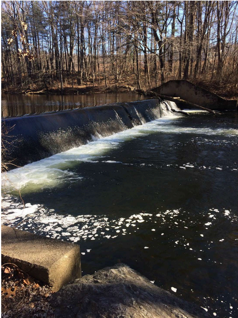
1. Dana Dam – The dam is a full barrier to migratory fish, and disrupts fluvial processes - including the transport of sediment to the estuary downstream.
