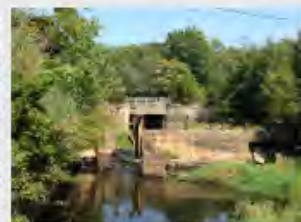
Cotton Gin Mill Dam, looking upstream.
