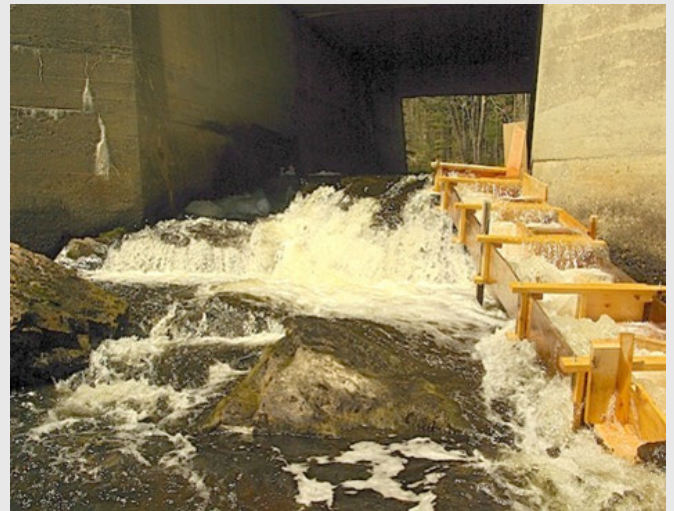
The Route 172 barrier on Patten Stream (facing upstream), with temporary fish ladder in place.
