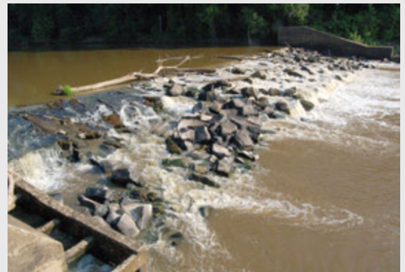
Lock and Dam 2. Native rock substrate was placed approximately 800 feet downstream.
