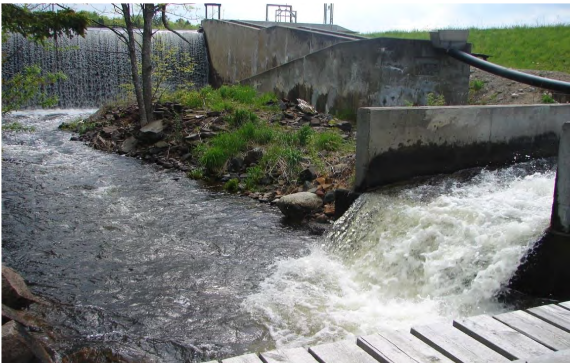
Figure 30. Dam and fishway under high flow conditions in 2006. Note harvest box and sluice pipe located at the corner pool of the fishway used to transport harvested fish into totes.
