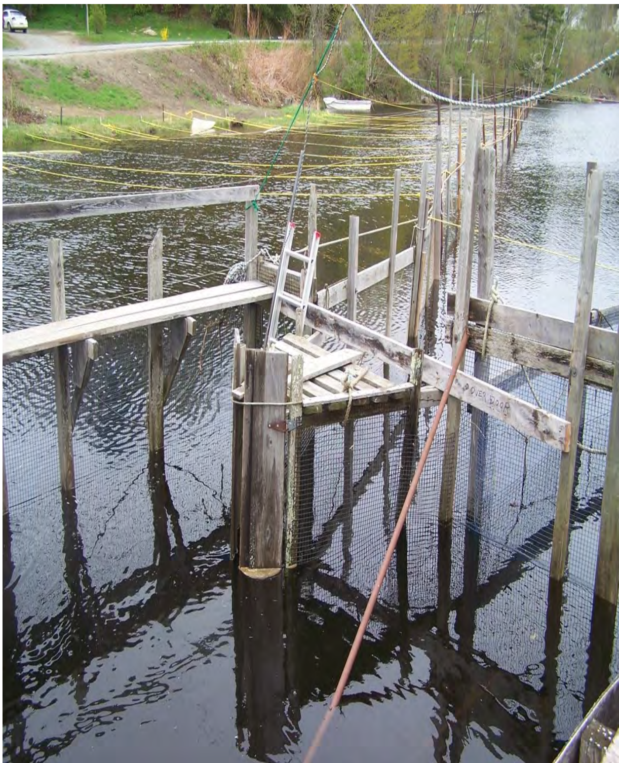
Figure 26. Fishing weir located at the head of tide on the St. George River in Warren, Maine.
