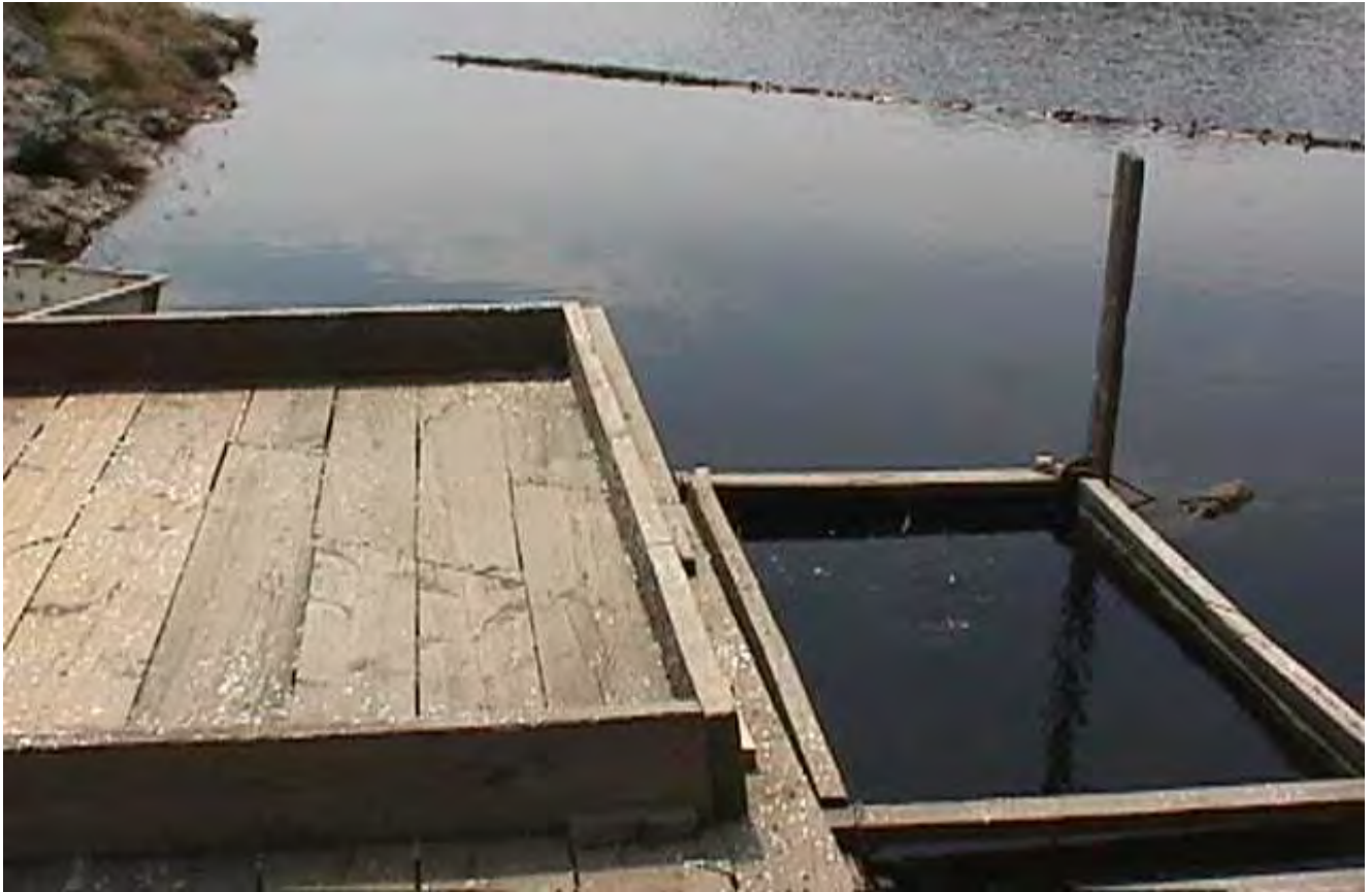
Figure 12A. The Winnegance fish trap located in the lake above the fishway.
