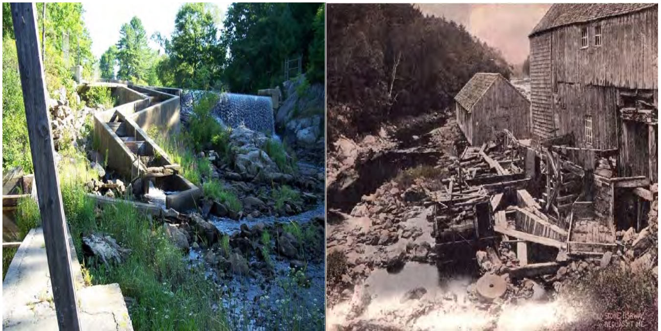
Figure 29. The Nequasset fishway and entrance to the trapping facility after repair in 2014.
