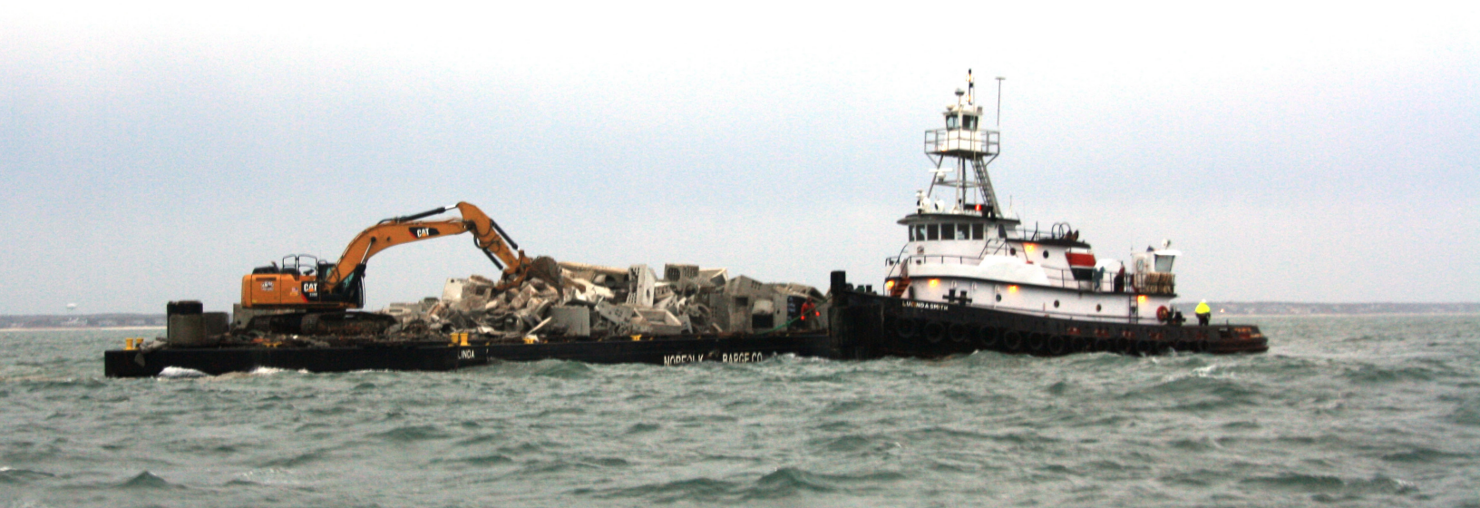
Figure 4. Deployment of materials to the Harwich Artificial Reef site. Photo credit: Mark Rousseau, MA DMF.
