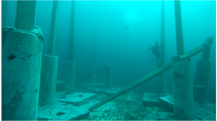
Figure 44. Reef darts that were deployed offshore Palm Beach, where some of the structures were damaged during deployment. Each structure is around 30 feet tall and was designed by a local fishing club.
