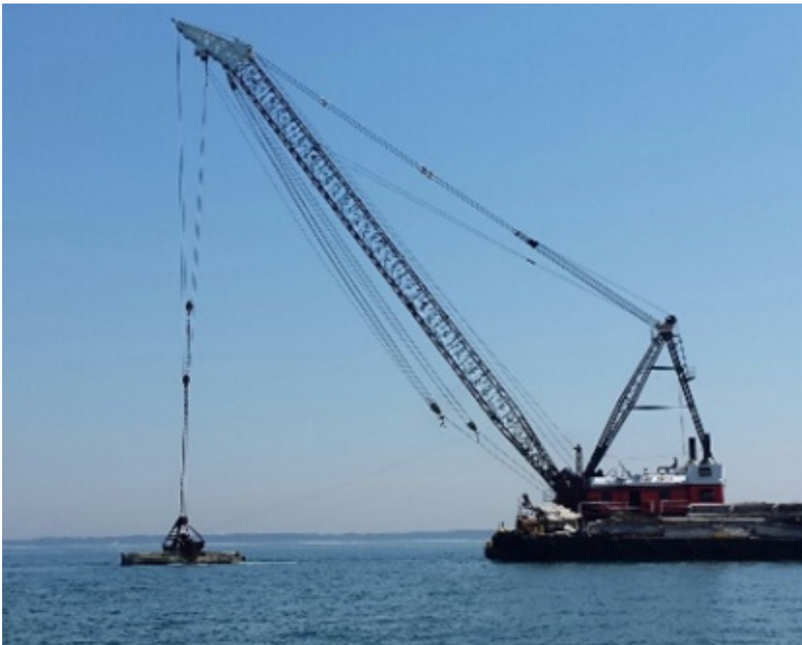
Figure 29. Deployment of Lesner Bridge material to the Cabbage Patch by McClean Contracting Company (2017). Photo credit: VMRC.
