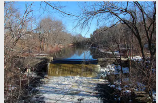
Coopers Mills Dam, Sheepscot River
