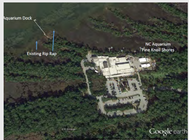
Aerial view of the project site
