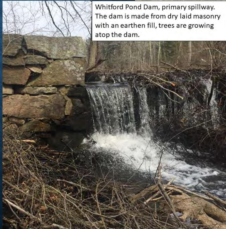
Whitford Pond Dam, primary spillway. The dam is made from dry laid masonry with an earthen fill, trees are growing atop the dam.
