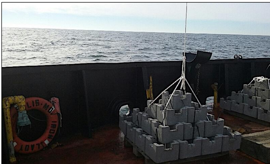
Figure 6. Oyster castle pyramids being deployed.
