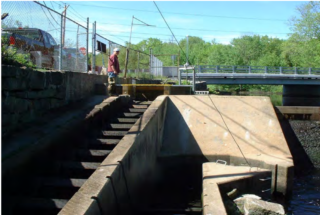
Figure 3: Photograph of the Potter Hill Dam and 1970's Constructed Denil Fishway with Fish Trap
