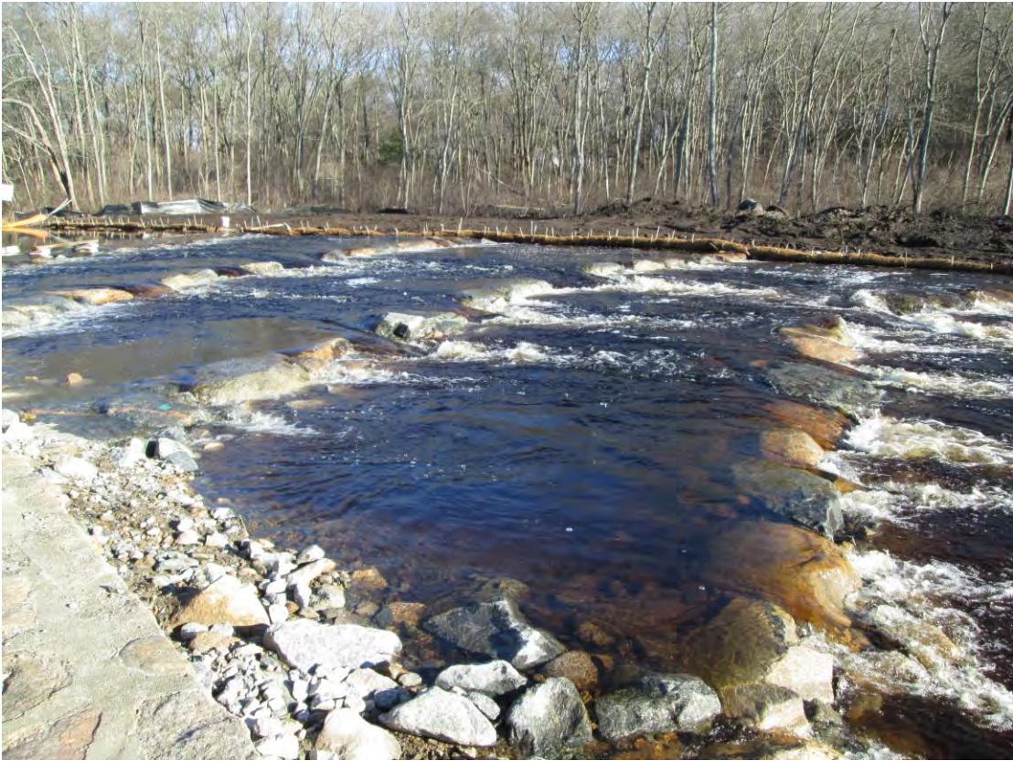
Figure 8: Construction of Rock Ramp Fishway at Kenyon Mill Dam
