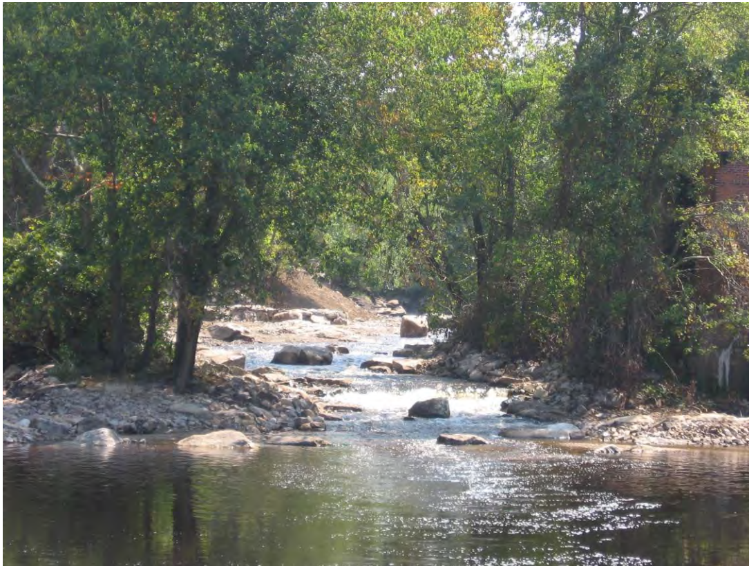
Figure 5: Photograph of Dam Removal and Rock Weirs at Lower Shannock Falls
