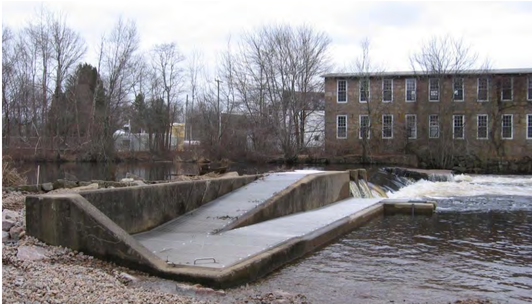
Figure 4: Photograph of the Bradford Dam and 1970's Denil Fishway
