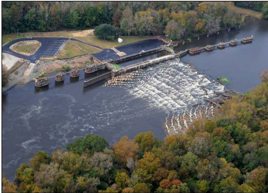
Figure C 50 – NLF installed in place of the Lock and Dam #1 on the Cape Fear River, NC completed in 2012. Credit: USACE.
