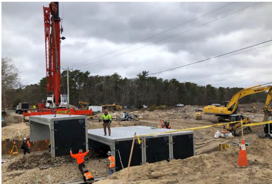
Figure C 11 – New, fish passage-friendly culvert installation at John Parker Road, May 2020. Credit: NOAA Fisheries.
