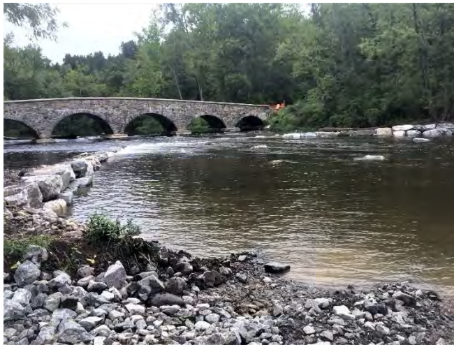
Figure C 31 - Brugler Bridge rock vane construction, view from downstream. Credit: Beth Styler Barry/ TNC.
