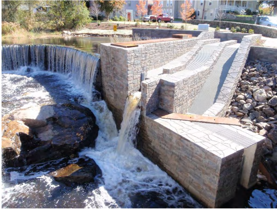
Figure C 25 – Horseshoe Falls dam with Denil fishway and eelpass, completed 2012. Credit: NOAA Fisheries.
