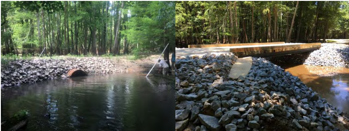
Figure C 47- Undersized culvert (before, left) and bridge (after, right) at Phase 3 location on Ware's Gut at the RTRGC property. Credit: Aaron McCall/ TNC.
