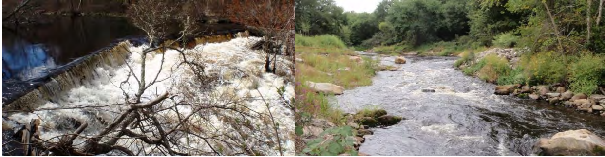
Figure C 19 – Lower Shannock Falls Dam removal. Existing dam (left – 2008) and river restored after dam removal (right – 2011). Credit: NOAA Fisheries.
