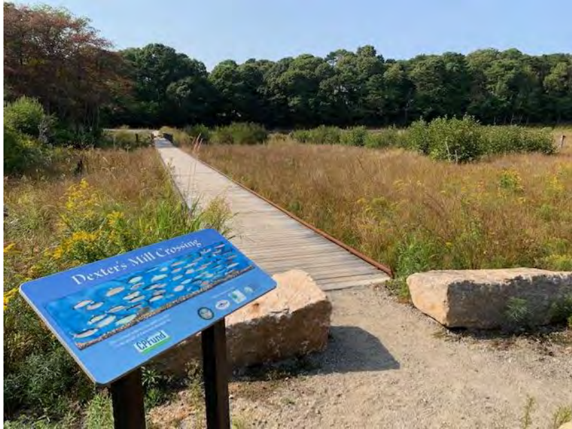
Figure C 10 – Dexter’s Mill Crossing boardwalk, site of former Lower Bog Dam. Dam removal site is in the background at bridge crossing. Wetland restoration at former cranberry operation. Credit: NOAA Fisheries.
