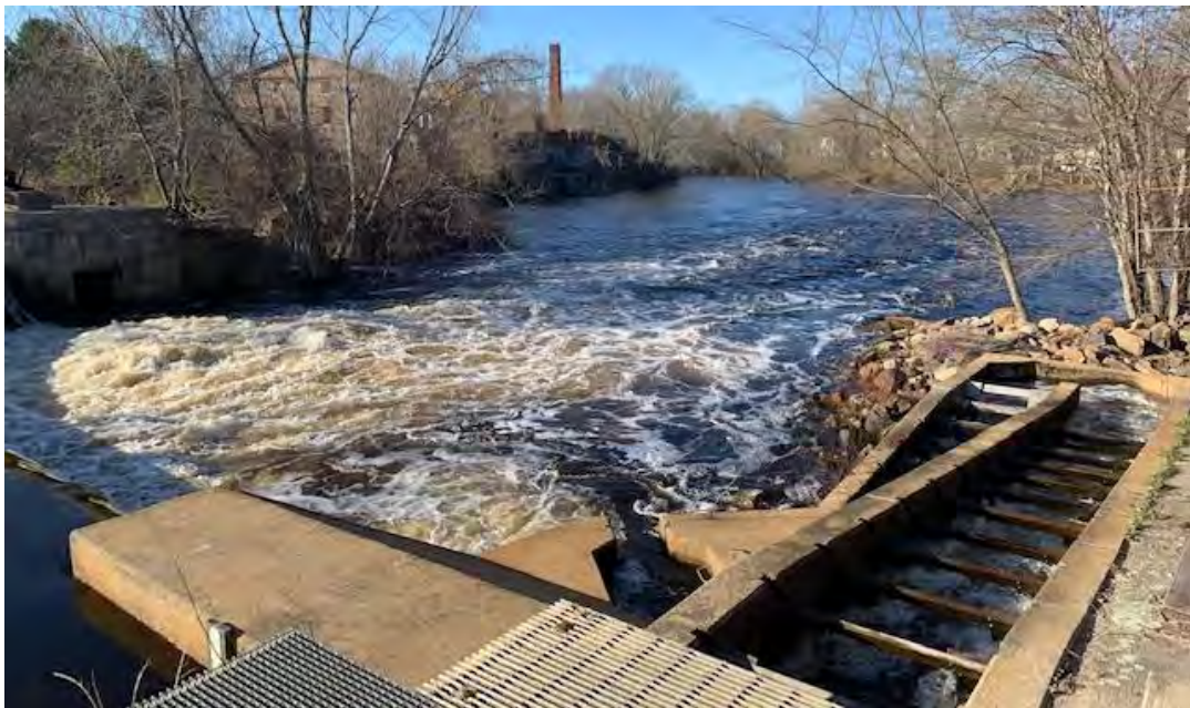
Figure C 26 - Potter Hill dam in April 2022. Narrow spillway encumbers excessive flows, creating broad hydraulic at toe of spillway. Existing fishway (circa early 1970s) functions poorly due to location of the entranceway (lower center of photo) and truncated operational flow range. The removal of the decrepit mill (background, river left) and last mainstem dam remain under consideration by the Town of Westerly and Rhode Island Superior Court in 2022. Credit: NOAA Fisheries.
