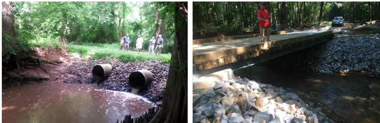
Figure C 45- Perched culverts (before) and bridge (after) at Phase 1 location on Ware's Gut at the RTRGC property. Credit: Aaron McCall/ TNC.
