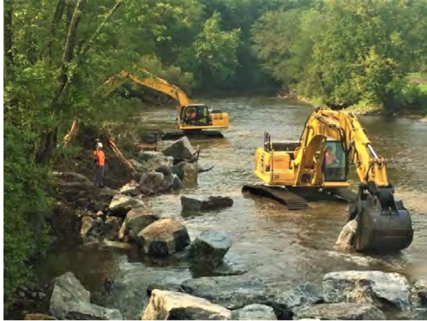
Figure C 30 - Brugler Bridge rock vane construction Credit: Beth Styler Barry/ TNC.
