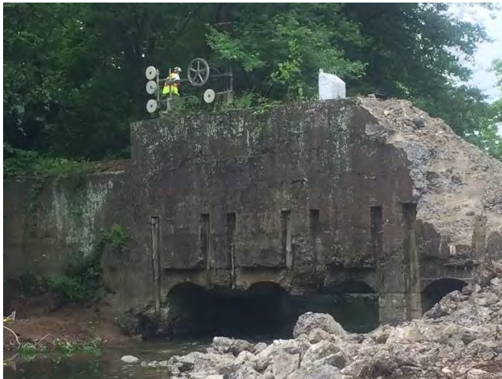
Figure C 29 – Removal of remnants from the Columbia Dam. Credit: Beth Styler Barry/ TNC.
