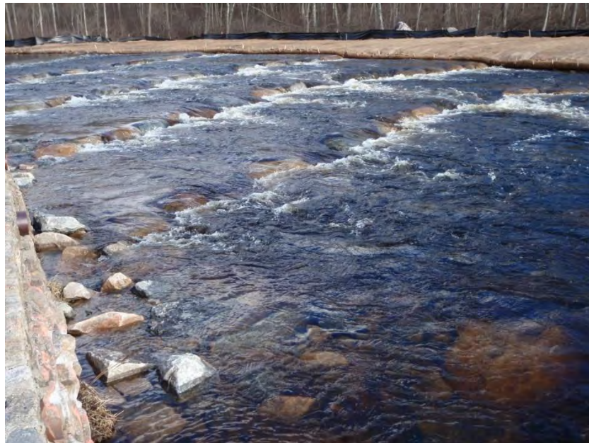
Figure C 21 – Kenyon Mill step-pool NLF, uppermost fish passage site, completed 2013. Credit: NOAA Fisheries.
