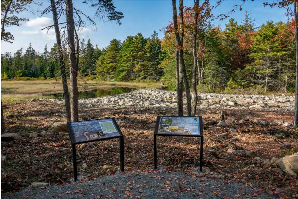
Figure C 4 – Meadow Brook rock ramp style NLF, equipped with public walking path and interpretive signage. Credit: Ken Woisard Photography/ MCHT.
