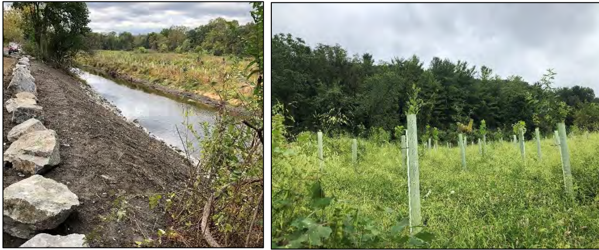
Figure C 33 – Road area streambank protection (left) and riparian plantings (right) including 10,000 trees, willow stakes and whips. Credit: Beth Styler Barry/ TNC.
