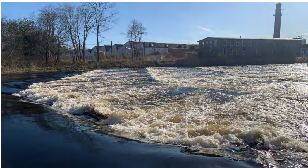
Figure C 23 – NLF at Bradford Dyeing site, spring flows, 2022. High fish passage flows have submerged the lower weirs, attributed to downstream backwatering. Credit: NOAA Fisheries.
