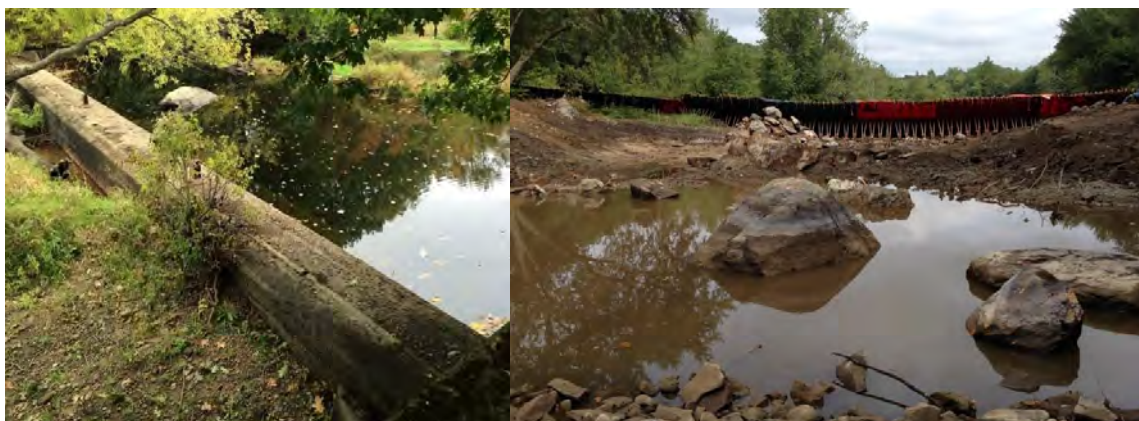
Figure C 18 – White Rock dam removal: Existing dam and accumulated sediment behind dam (left) and dam removal with upstream port-a-dam to divert flows into raceway, October 2015. Credit: NOAA Fisheries.
