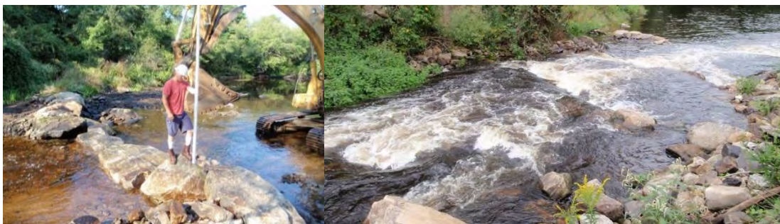
Figure C 24 – Modification of the backwatering weirs downstream of Lower Shannock Falls Dam removal to improve passage efficiency (left – 2011) and view of the backwatering weirs during low fish passage flows (right – 2012). Credit: NOAA Fisheries.
