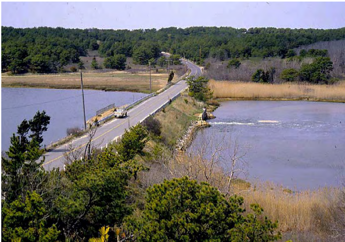
Figure C 15 – Current Chequessett Neck Road Bridge and culvert structure. Credit: National Park Service.
