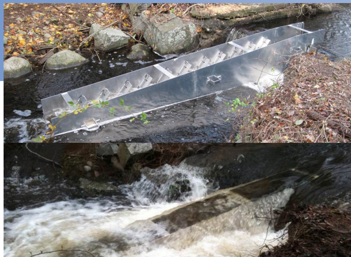
The Vargas Pond fishway on Stony Brook in Stonington, CT, illustrating the very different passage conditions that can exist under both low flow (top) and high flow (bottom) conditions. Source: CT Dept. of Energy and Environmental Protection, Inland Fisheries Division
