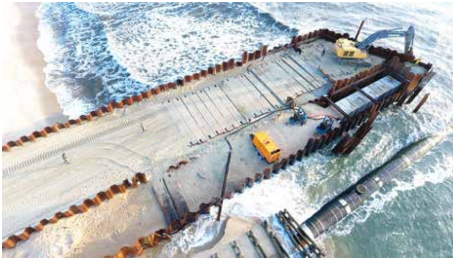
The bypass culvert. Photo credit: The American Littoral Society
