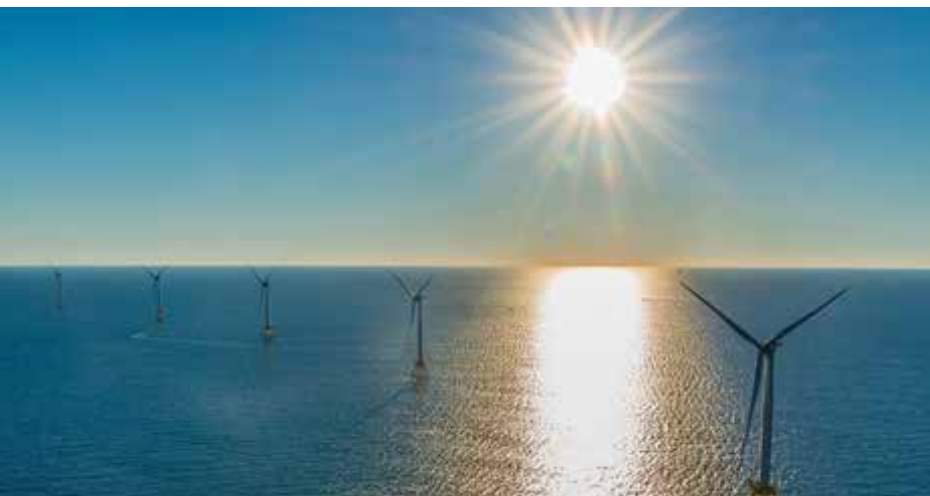
The Block Island Wind Farm following completion in August 2016. Photo credit: Deepwater Wind, LLC
