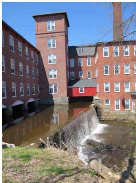
Right: Sawyer Mill Dam, Dover, NH Photo Credit: Kevin Lucey (NHDES, Coastal Program)
