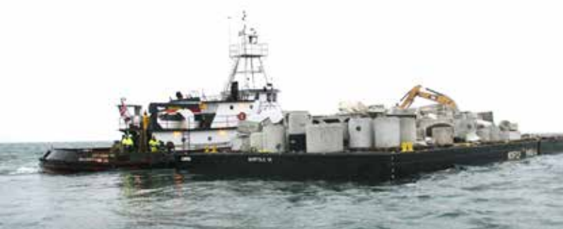
Concrete rubble being transferred to create the new Harwich artificial reef. Photo credit: Mark Rousseau, MA DMF
