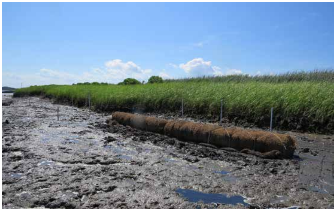
A coir log treatment for the SCDNR living shoreline study in coastal South Carolina. Photo credit: SCDNR
