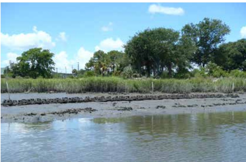
Overlook Park, Brunswick, Georgia: Deployment of 100 oyster balls placed on top of 25 double wooden pallets banded together. Bags of recycled oyster shells were also used to fill free spaces on top of pallets. Photo credit: January Murray, GA DNR
