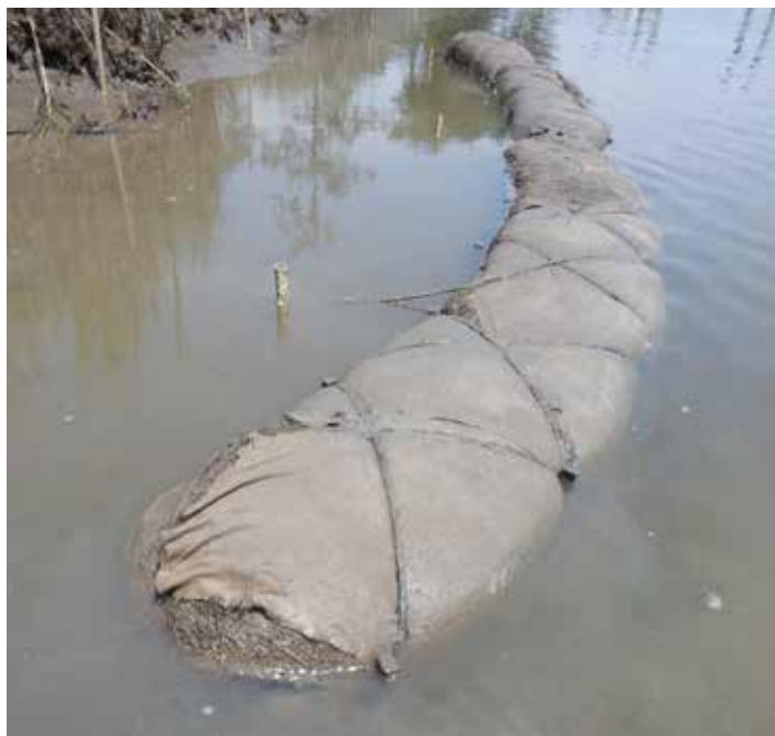
A Curlex® fiber treatment for the SCDNR living shoreline study site in coastal South Carolina. Photo credit: SCDNR
