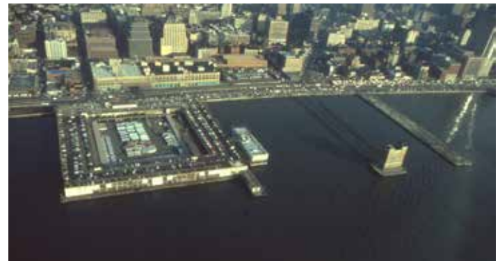
Figure 3. Manhattan shoreline showing typical man-made structures (piers, pile fields) constructed over filled in areas near shore. Used with permission from Dr. Ken Able, Rutgers University
