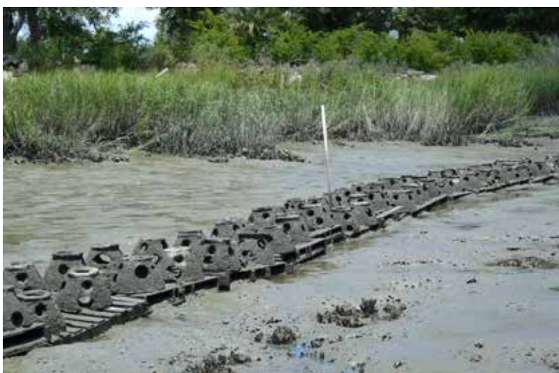
Overlook Park, Brunswick, Georgia: Deployment of 100 oyster balls placed on top of 25 double wooden pallets banded together. Bags of recycled oyster shells were also used to fill free spaces on top of pallets. Photo credit: January Murray, GA DNR
