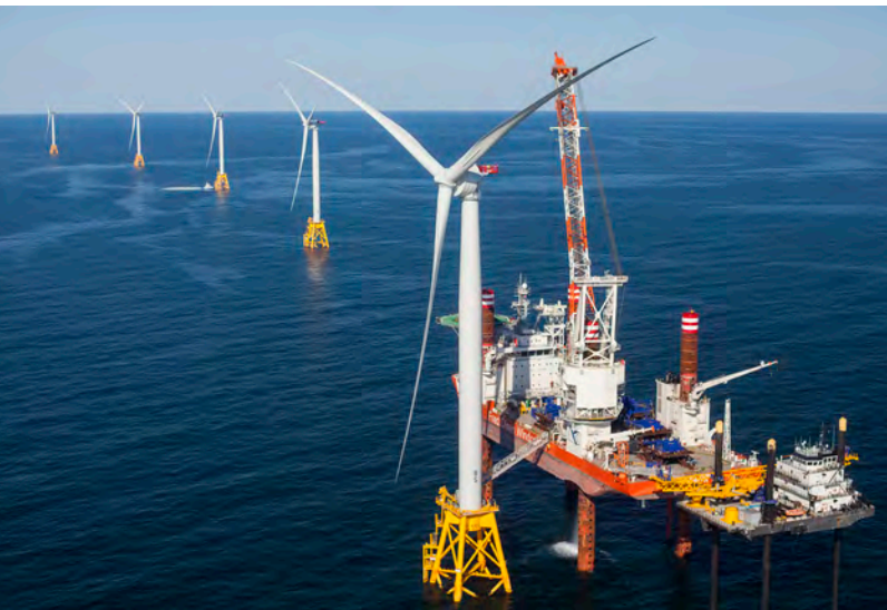
Block Island Offshore Wind Farm, Rhode Island (Deepwater Wind). Image credit: American Wind Energy Association.
