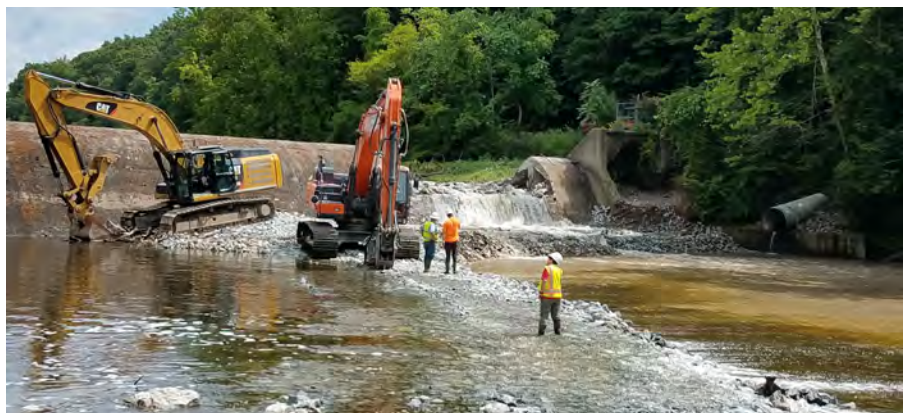
Crews remove an obsolete dam within the Columbia Wildlife Management Area to restore access for migrating fish to their historic spawning grounds. Image credit: NJDEP.
