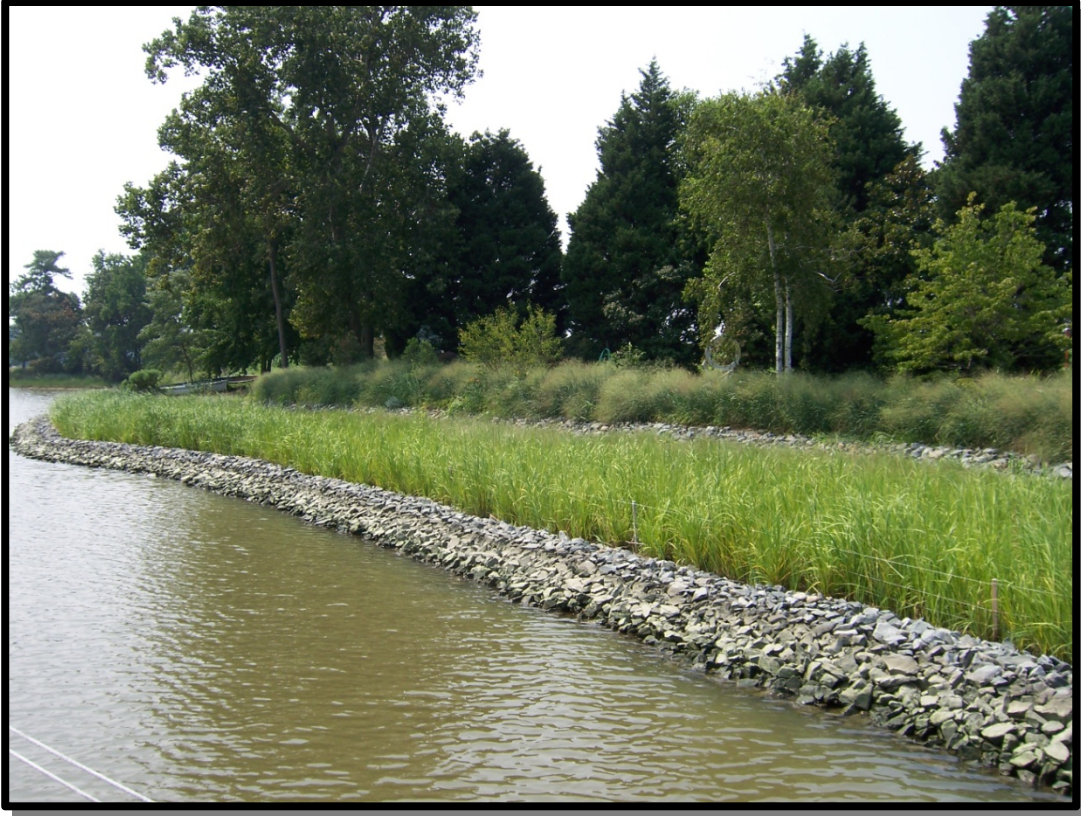
Figure 19: Example of a living shoreline in Maryland (Photo credit: Maryland Department of Natural Resources)
