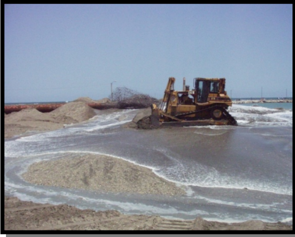
Figure 4: Renourishment with heavy equipment (Photo credit: Florida FWC)
