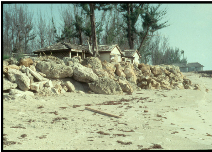
Figure 10: Sloped beach revetment made of native limerock (Photo credit: Florida FWC)
