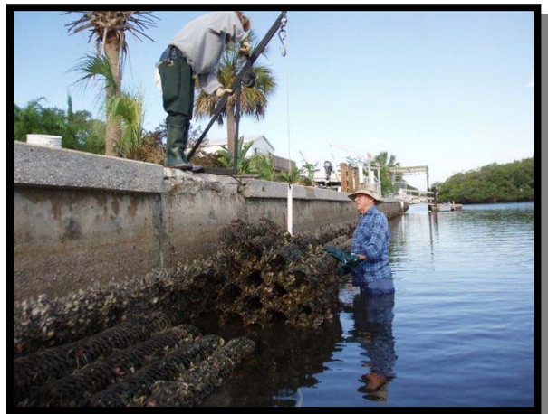
Figure 5: Concrete seawall with oyster settlement structures placed at the base (Photo credit: Florida FWC)
