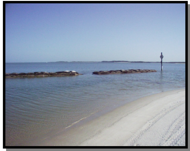
Figure 11: Concrete bag breakwater offshore of a sand beach (Photo credit: Florida FWC)
