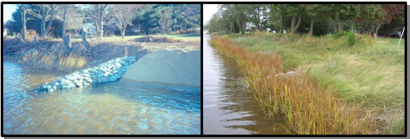
Figure 22: Example of pre (left) and post-installation (right) of a living shoreline in Maryland (Photo credit: Maryland Department of Natural Resources)
