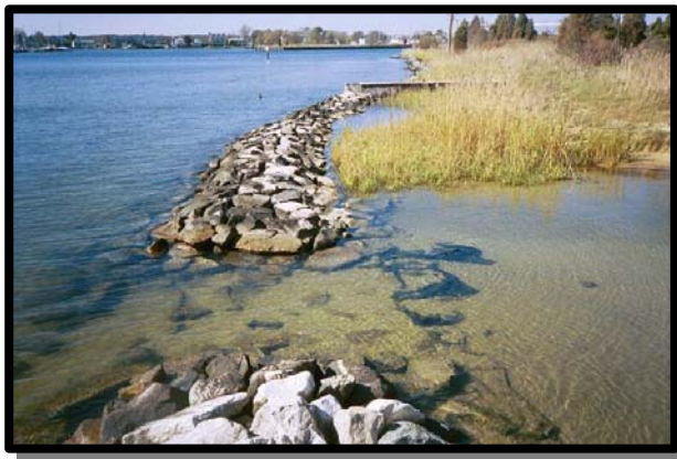
Figure 23: Example of a hybrid hard-soft shoreline stabilization (Photo credit: Maryland Department of Natural Resources)
