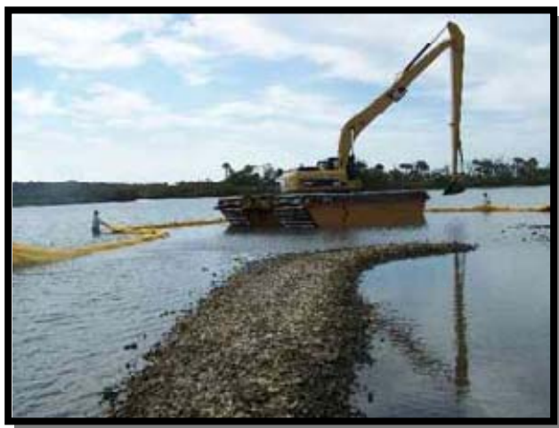
Figure 14: Oyster reef sill in the Mosquito Lagoon, Florida (Photo credit: Florida FWC)
